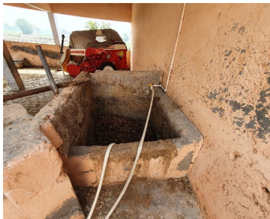
Domestic Bio-gas plant inlet
